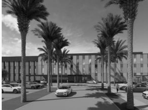
HonorHealth Medical Campus at Peoria will encompass 100,000 square feet. Image courtesy of Anchor Health Properties
